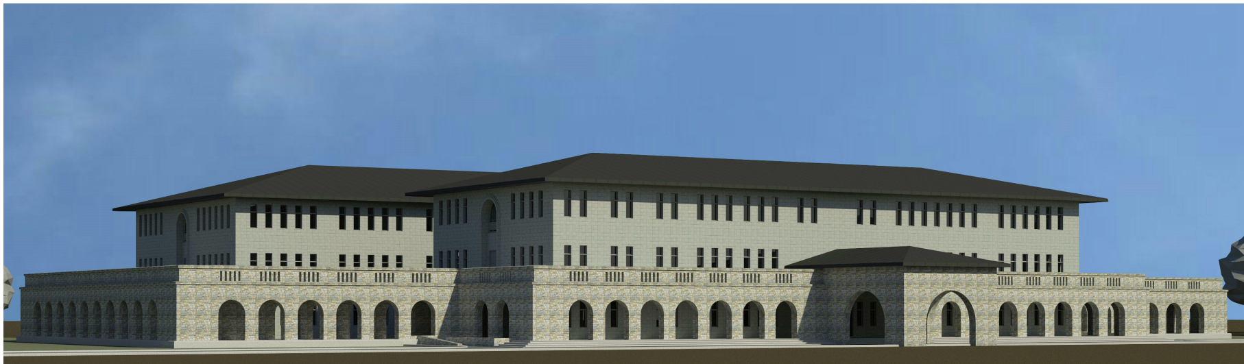
Structural Designs and Preparation of Estimates of Polytechnic College at Bethamcherla ,Nandyal Dist., A.P (Year 2022-23)
