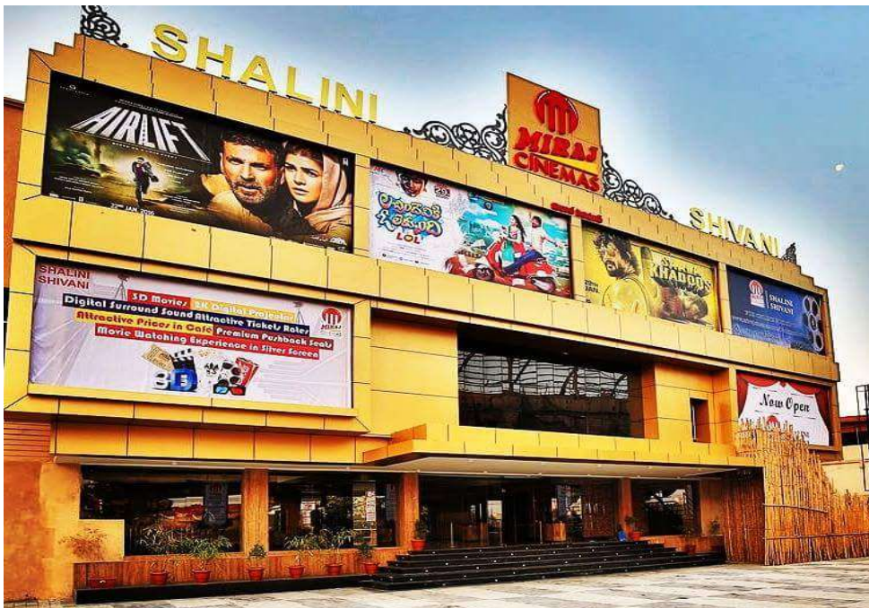
Construction of Civil and Structural works for 4 Screen Multiplex at Shalini & Shivani Theatre near Kothapet, Hyderabad (Year 2015-16)
