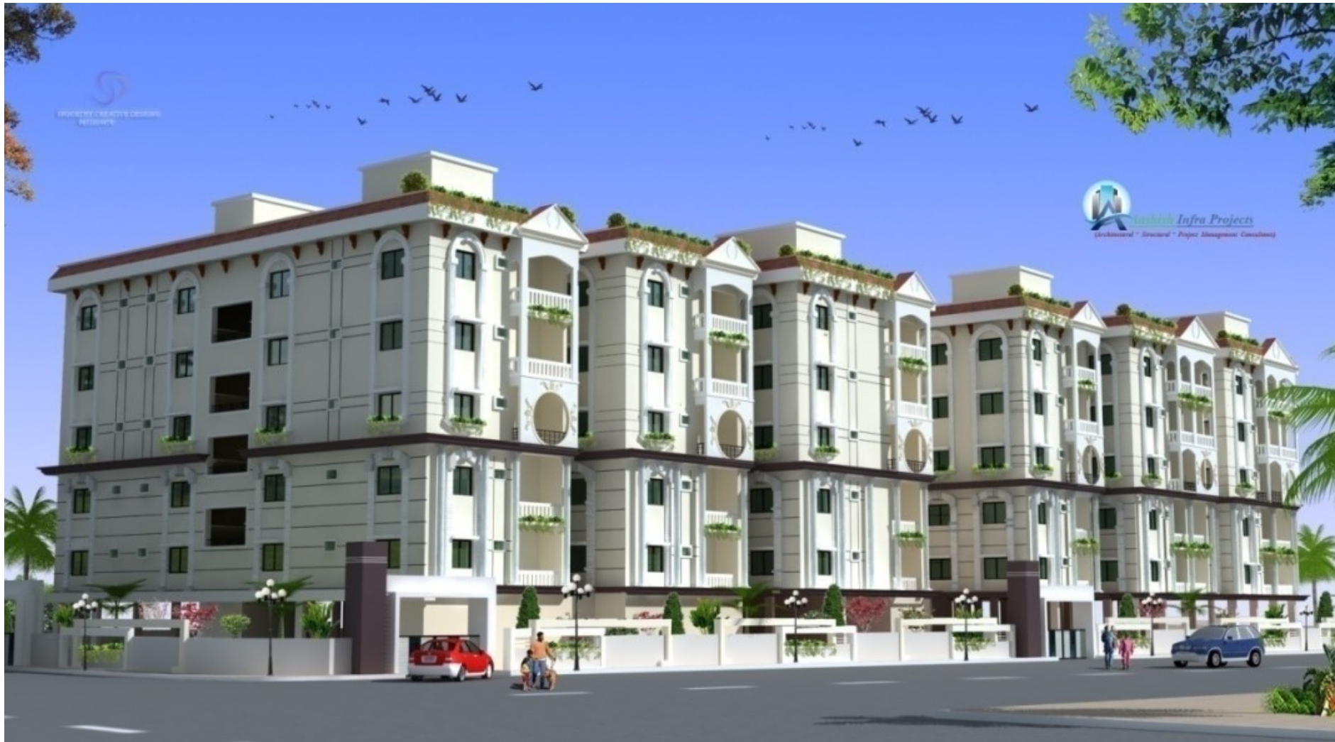
Construction of Residential (2 Cellars + 5 Upper Floors) at Budvel (Vi), Rajendra Nagar, Hyderabad.
