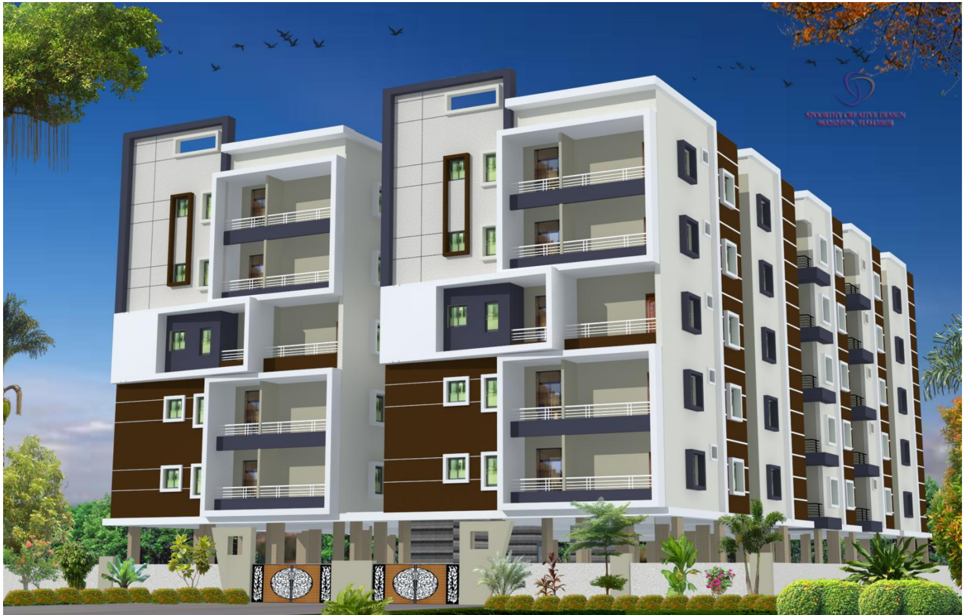
Planning and Designs (Arch., Structural & MEP) for Residential Apartment at Rayachoti, A.P (Year 2021-22)
